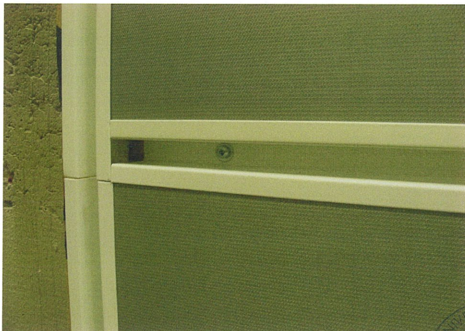
Photo 2 Tested elements detail: wall panels solution Rockfon VertiQ with Omega profile
